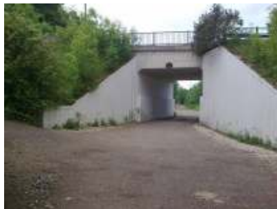
Proceed through Renishaw Tunnel
