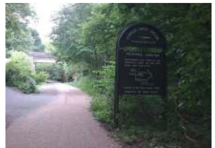
Thurgoland Tunnel ahead with new Trail surface
