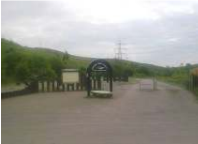
Entrance to the Trail at Dunford Bridge
