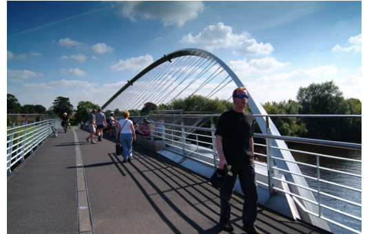
Millennium Bridge, York
