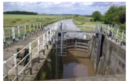
Cross over the Weighon Lock by the River Humber
